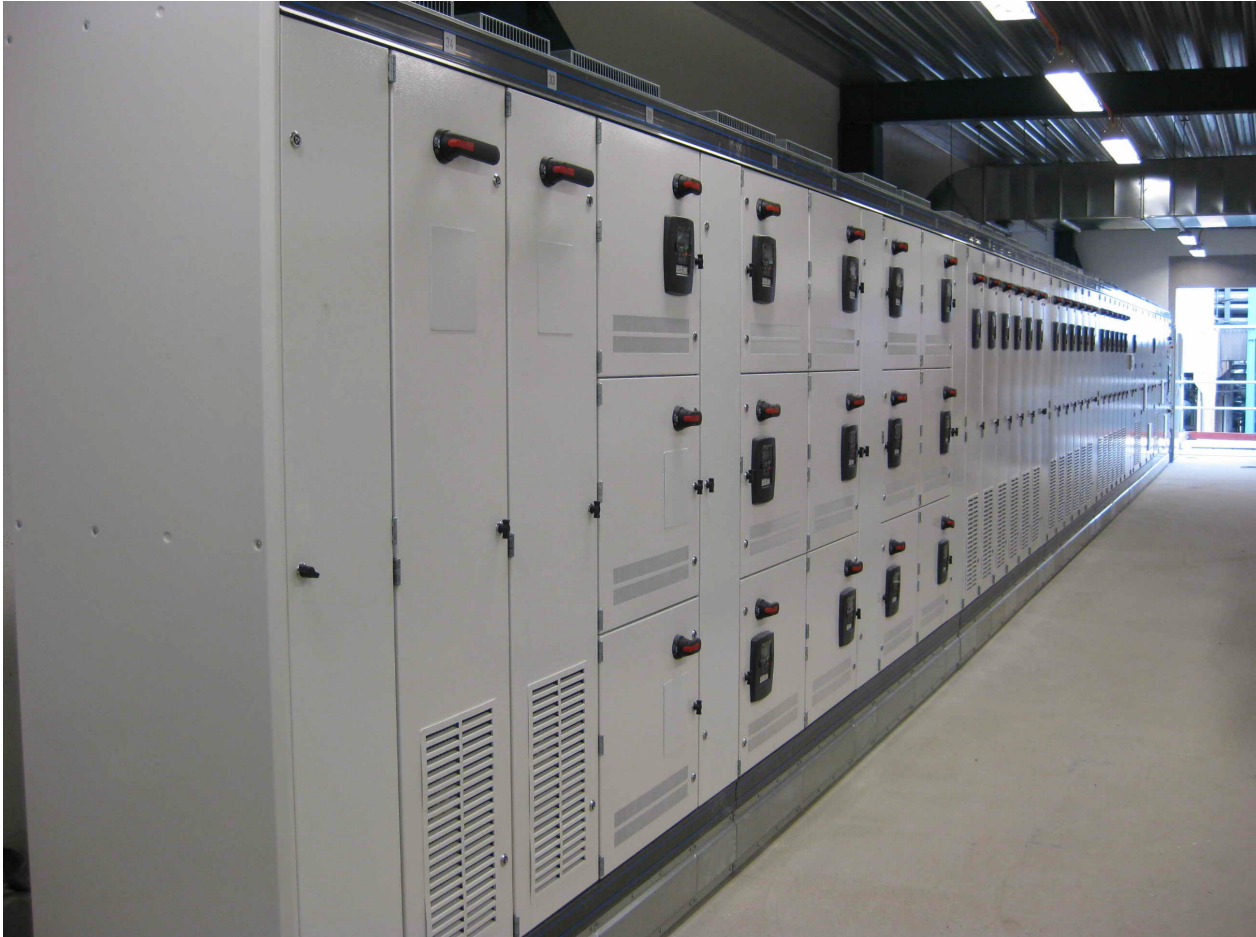
Figure 3. A common DC bus line-up
