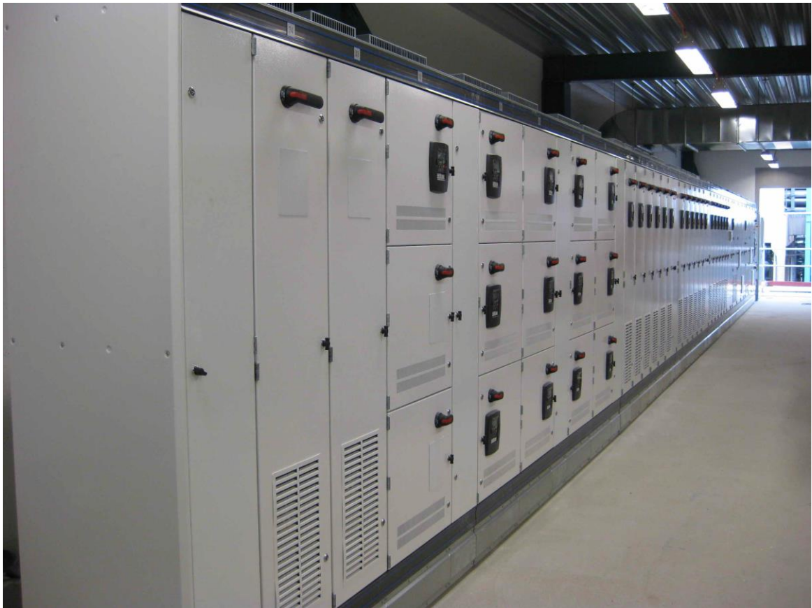
Figure 3. A common DC bus line-up
